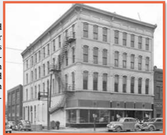
Goodwill Retail store and Work Evaluation Center at 601 Cherry St. It was named the Morral building in honor of William W. Morral who donated $10,000 to Goodwill in 1938.
